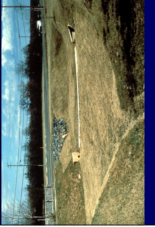
Typical Dry Detention Pond, with Pilot Channel
