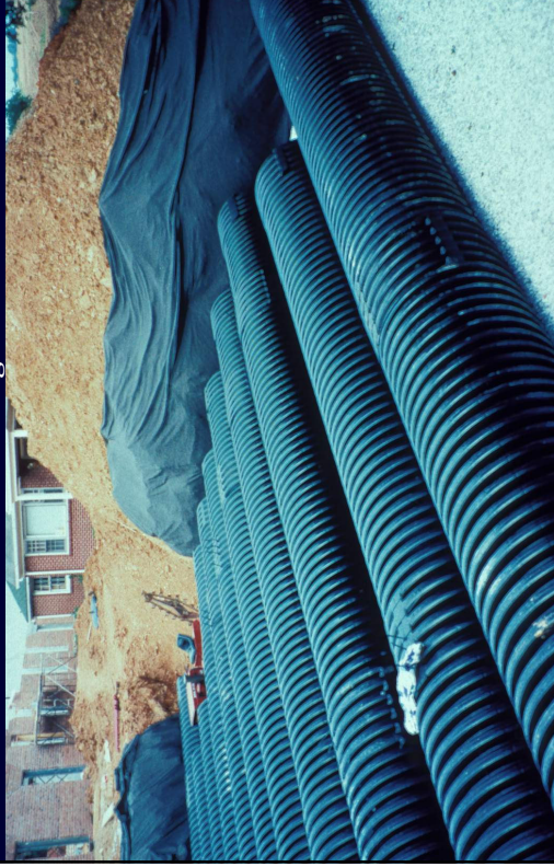
Large Corrugated Pipes used for Underground Detention Below Parking Area
