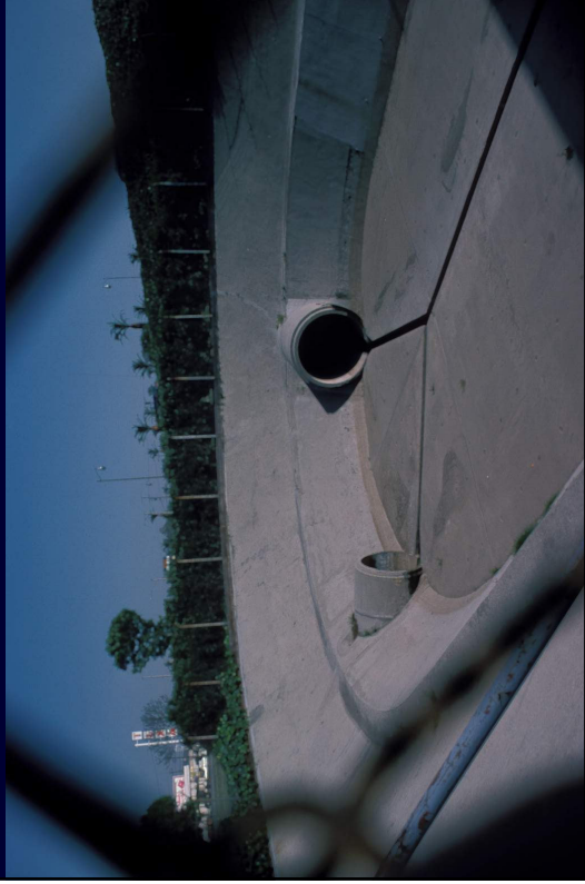
Dry Detention Pond Forebay for Stormwater Pump Station, Los Angeles, CA
